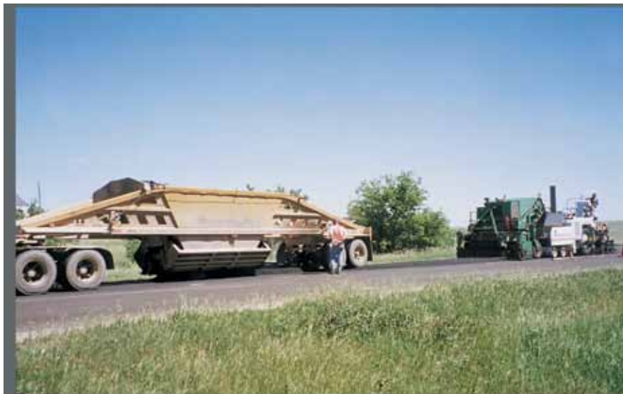
BOTTOM DUMP TRAILER DISCHARGING WINDROW
