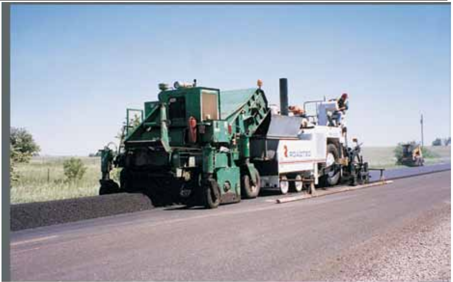
WINDROW PICK-UP MACHINE ON PAVER
