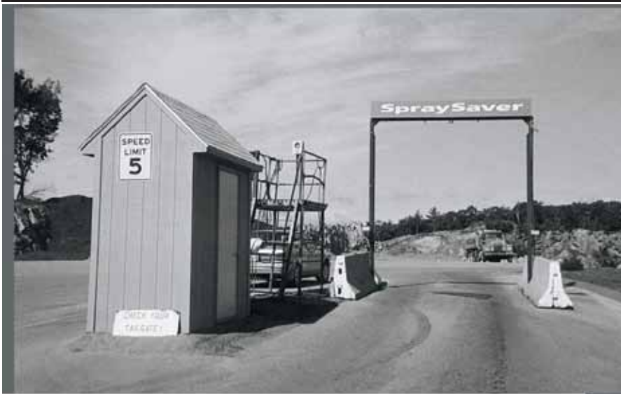
RELEASE AGENT APPLICATION SYSTEM
