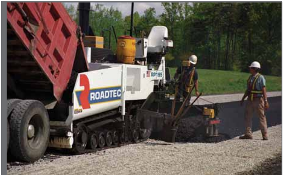
CONTROL THE HEAD OF MATERIAL TO ± ONE INCH
