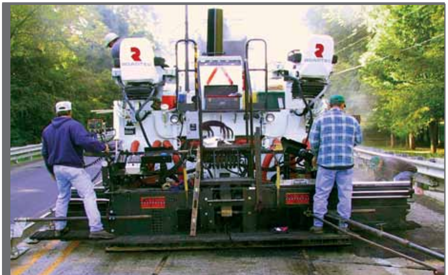
SETTING UP THE SCREED TO ACHIEVE GOOD TRANSVERSE JOINT
