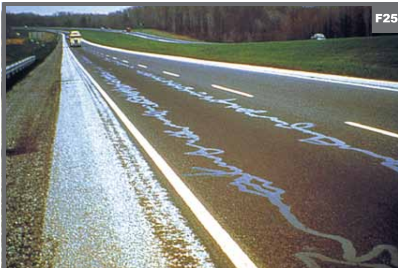
Rutting Often Occurs in Older Overlay Pavements
