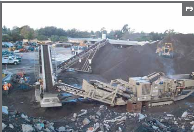
RAP Crushing Plant
