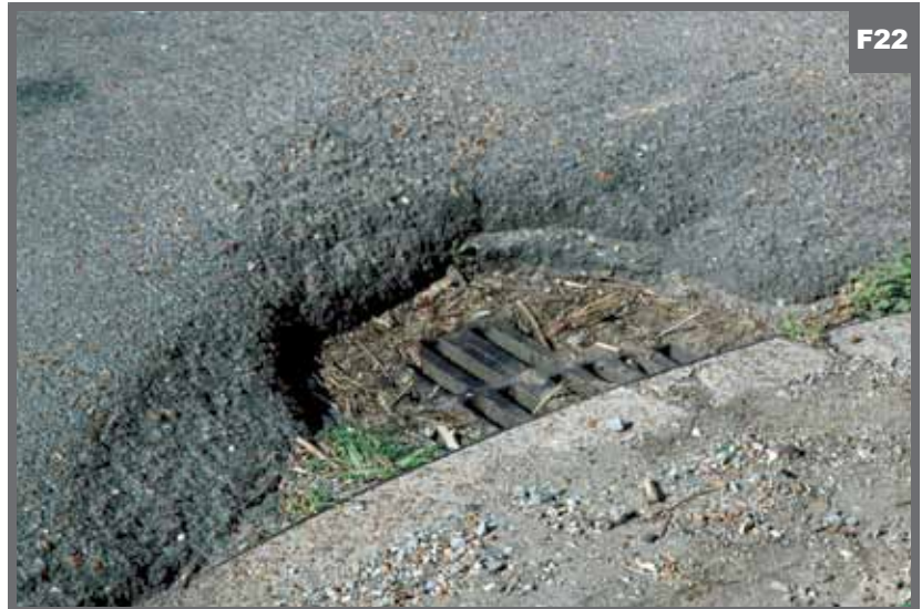
Multiple Overlays Create Drainage Problems
